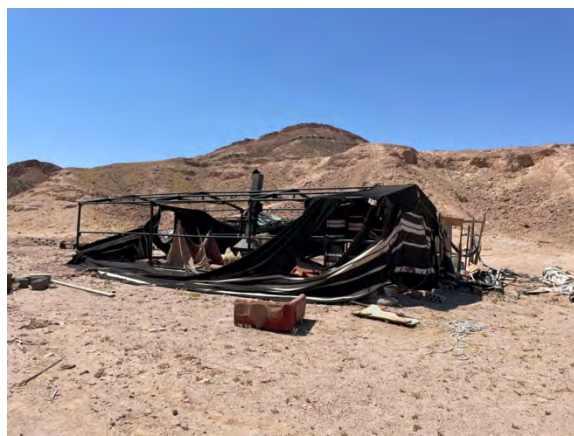
Abandoned Deteriorated Structure
