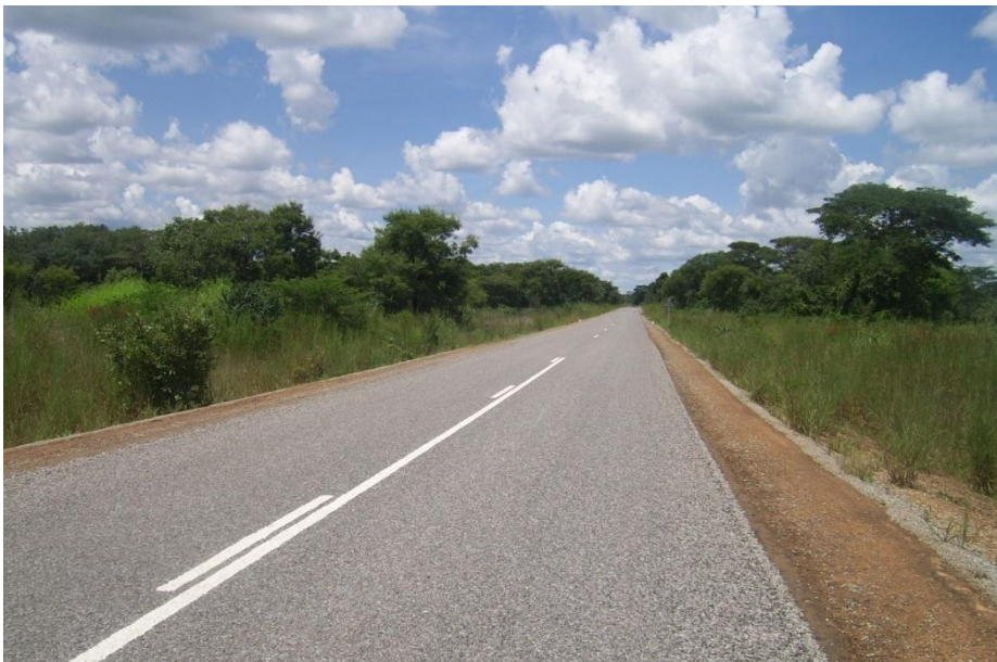
Figure 7: A section of the newly tarred road between Kasempa t-off and Mufumbwe
