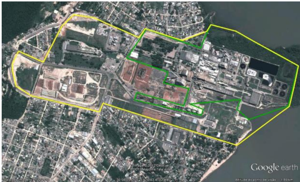
Figure 2.1. Aerial view of the Guaíba 2 mill site indicating current extent of the existing line 1 (in green) and the mill boundary after the expansion (in yellow).
