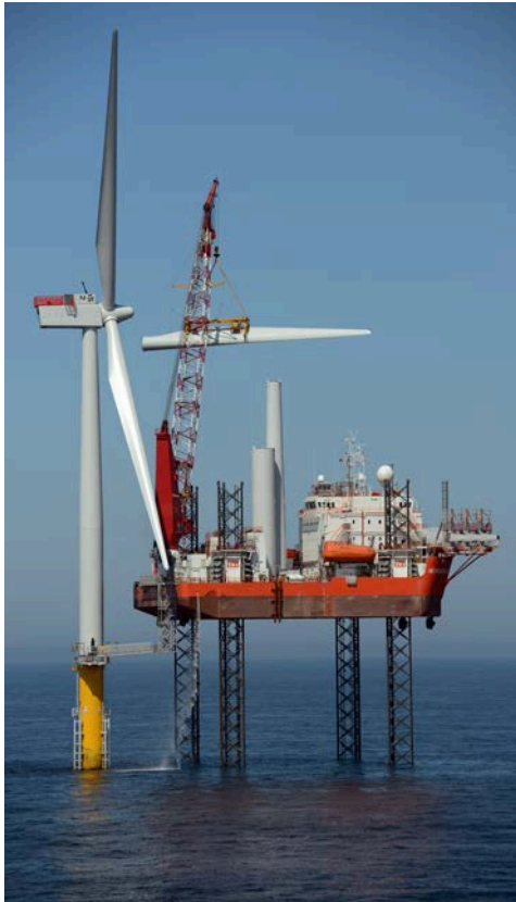
Offshore turbine construction
