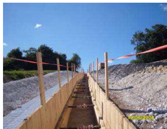
Onshore cable trenching
